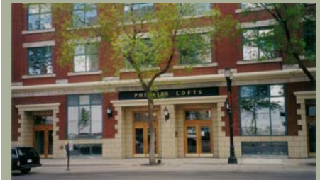
Phillips Lofts, residential re-use of an historic building
